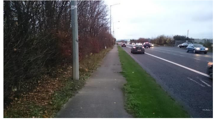
VIEW EASTWARDS ON APPROACH TO PROPOSED SITE ACCESS ON R139
